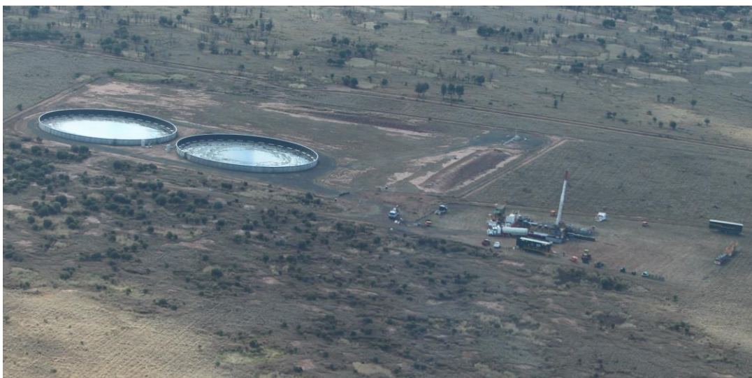
Figure 3 – Mira 5 under-reaming operations with the Mira pilot water storage tanks nearby.
