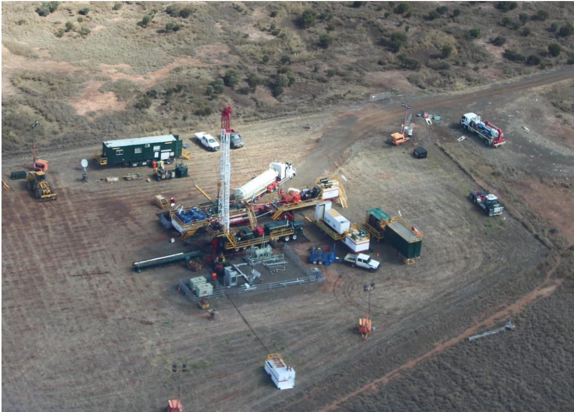
Figure 4 – Mira 5 under-reaming operations just before rig release on Monday 7 August.
