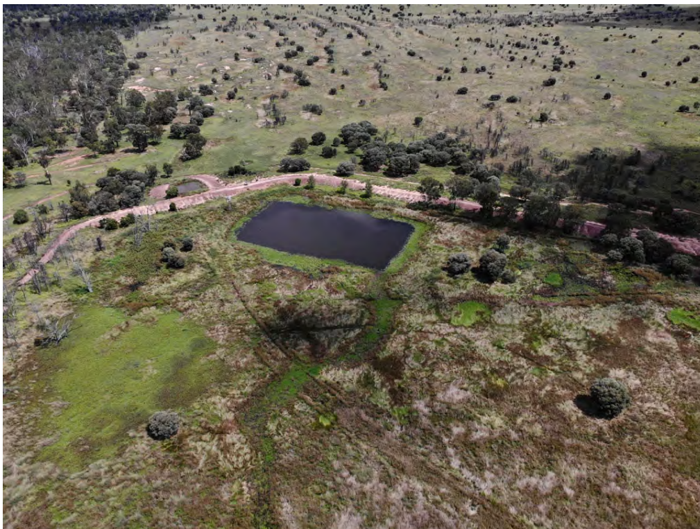
Aerial photograph from 100 m above ground level; upstream (left) to downstream (right)
